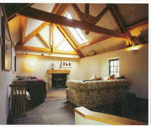
recycled and new stone. New blockwork was used when extra stability was required. A new roof was built from local Douglas fir timber trusses, which have been left exposed in the interior. Corrugated steel covers the roof externally, and several roof windows let extra daylight in.
